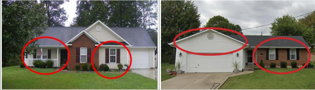
Figure 1204.06-2 Unacceptable Use of Vinyl
