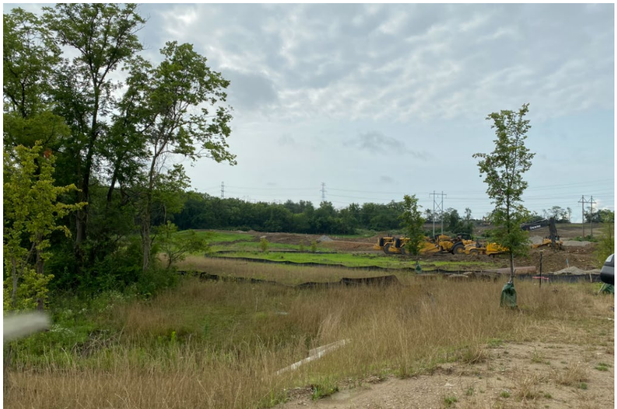
Facing South on Hanford Lane
