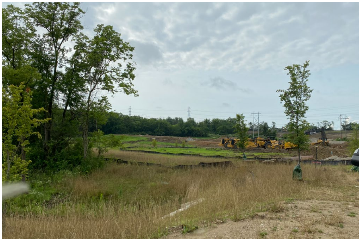
Facing South on Hanford Lane
