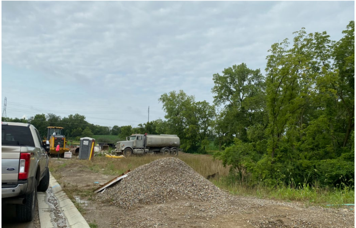
Facing South on Hanford Lane
