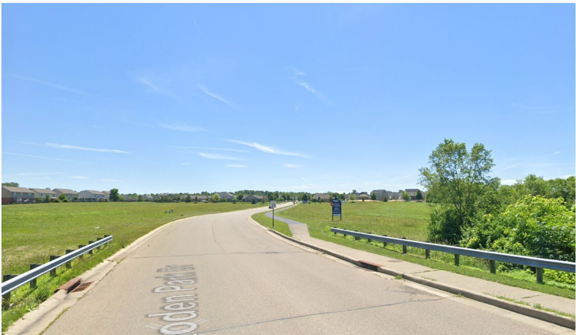
Eastbound on Roden Park Dr
