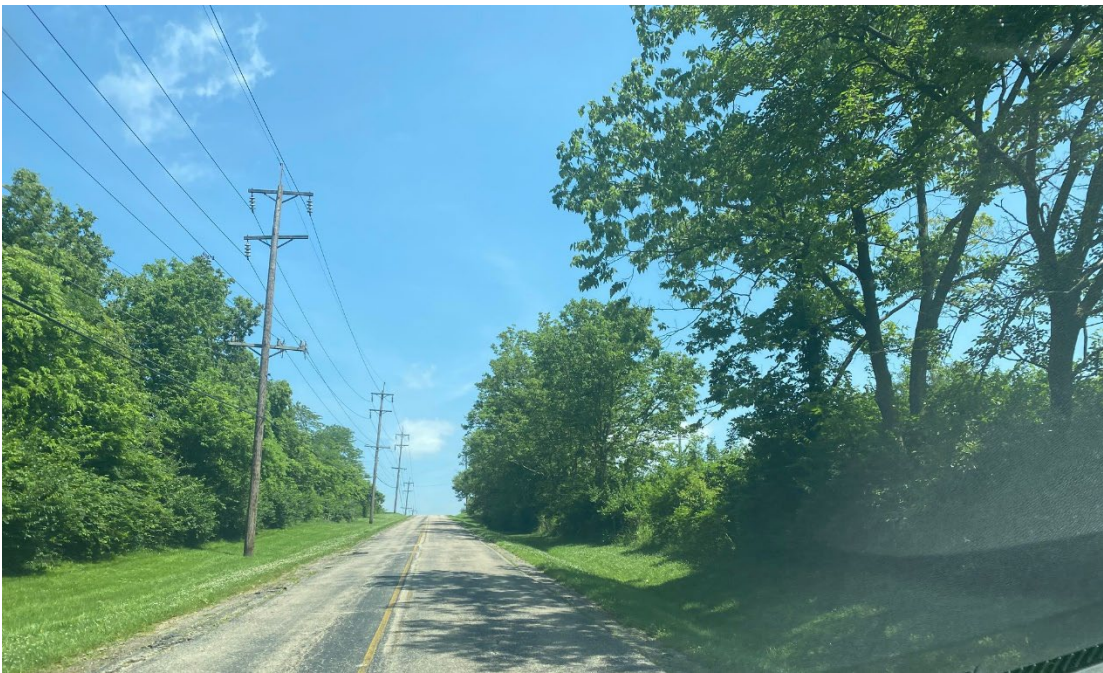
Northbound on Access Drive
