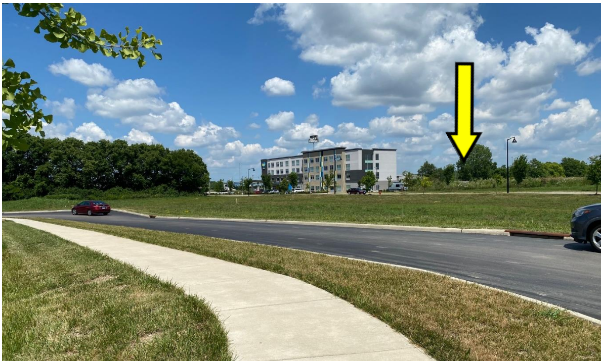
Facing Northwest at Private Drive
