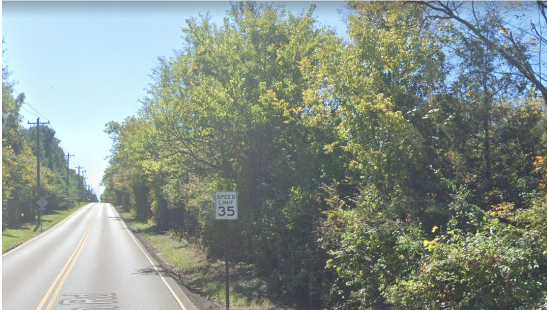
Southbound on Butler Warren Road
