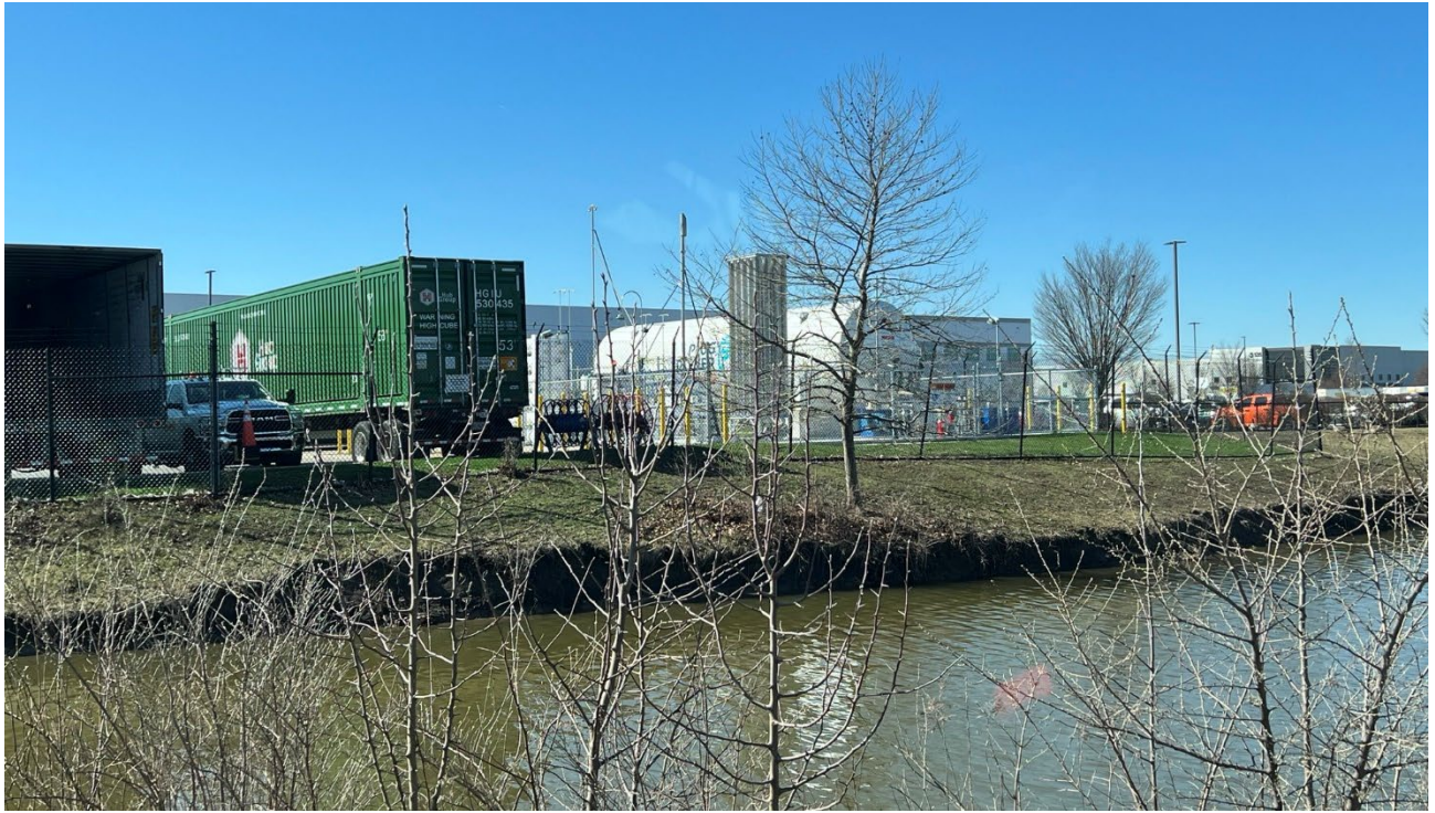
Looking southwest towards the hydrogen fuel area from Union Road
