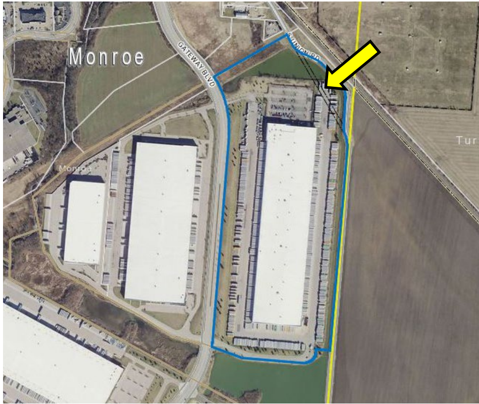
Overhead View of Site
