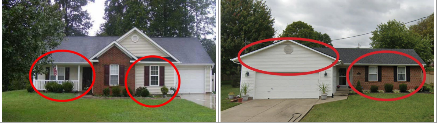
Figure 1204.06-2 Unacceptable Use of Vinyl
