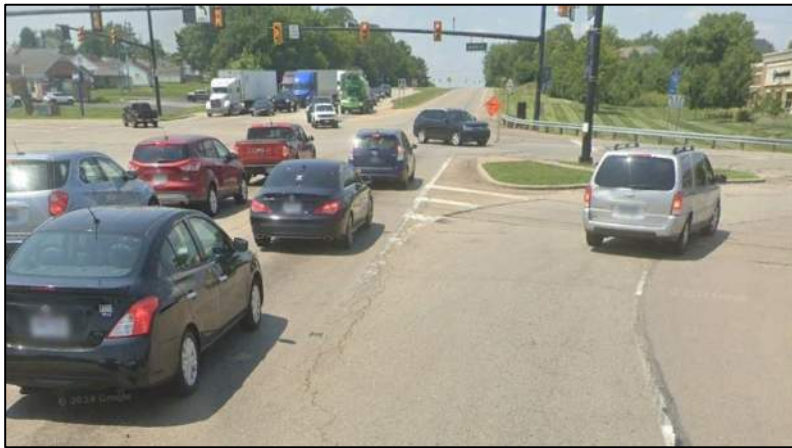
Photo 5: Westbound Right Turn Slip Lane with Worn Pavement Markings
