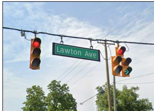
Photo 9: Signal Heads on Lawton Avenue
