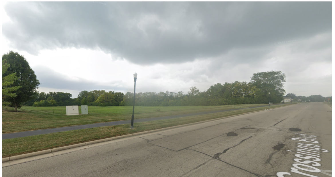
Northbound on Crossings Boulevard
