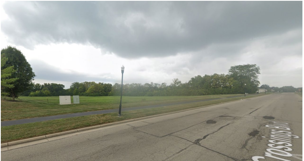
Northbound on Crossings Boulevard
