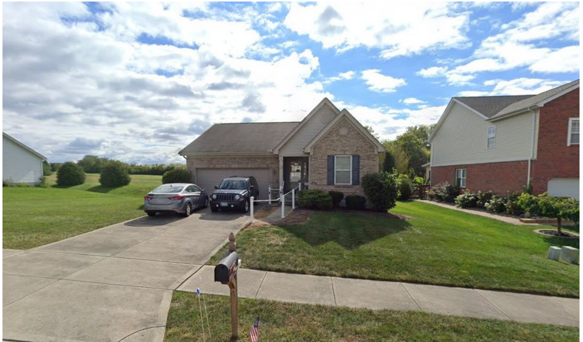
Looking Southwest towards the home from Bayberry Ln
